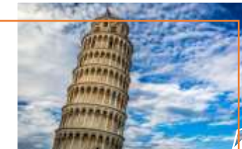
Leaning Tower of Pisa
